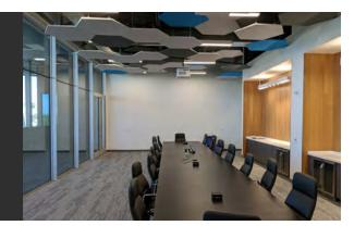
Made with a rigid fiberglass core and edge-hardened, these panels are wrapped with a variety of acoustic fabric colors and have tailored corners. They are ideal for spaces like conference rooms, auditoriums, meeting halls, or anywhere sound absorption is needed.
